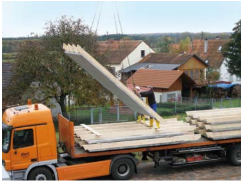
1. Delivery of the prefabricated solid roof elements
